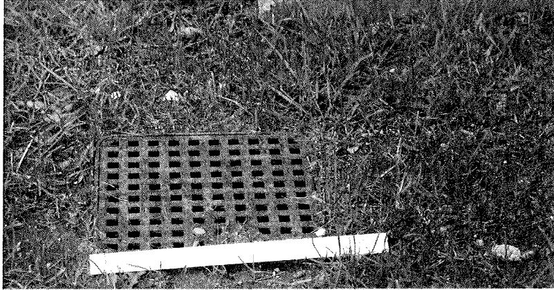
Inlet Capture Rate (m 3 /s) for Grate Small Grid inlet ( on Sag) and Curb and Gutter Type B
