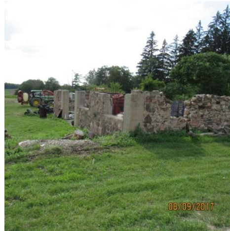
Plate 8: Stone barn foundation in farmscape, looking northwest.
