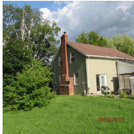
Plate 10: North and west elevations of the residence at 11490 Bathurst St.
