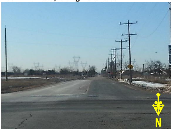
5. View of the rail crossing located south of the Phase One Property at McGillivray Road, facing south.
