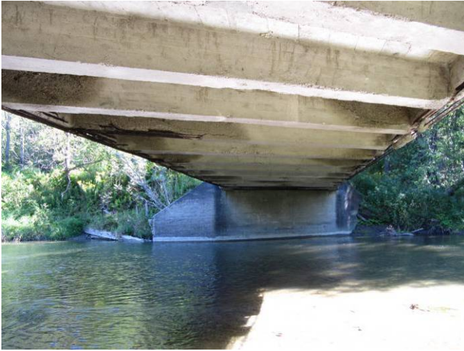
Plate 7: View under the bridge, looking east from the west abutment.
