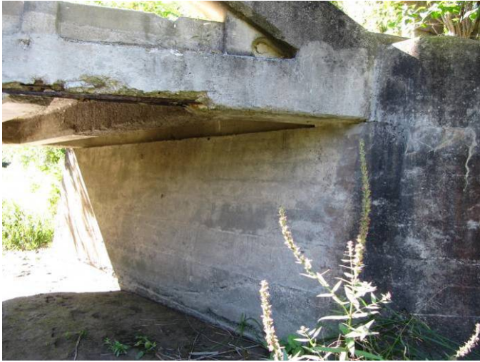
Plate 10: View of west abutment from the north.
