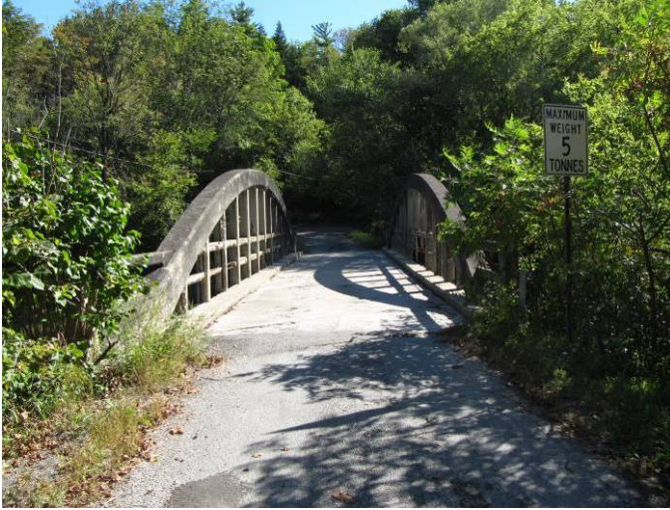
Plate 1: View of bridge crossing from the west.
