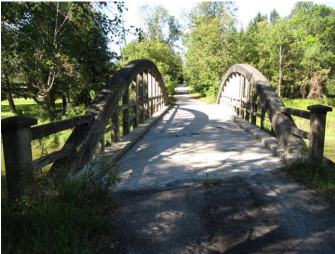
Plate 2: View of bridge crossing from the east.
