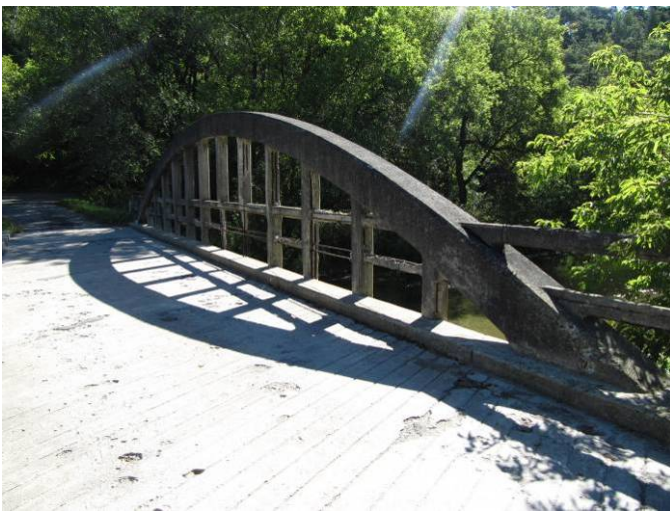
Plate 14: View of the south truss.
