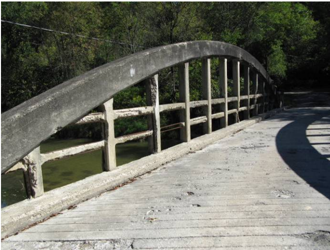
Plate 13: View of the north truss.
