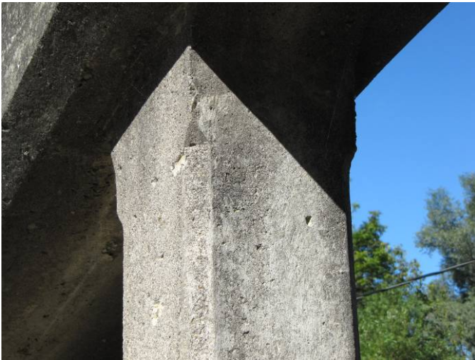
Plate 17: Detail of chamfered edges.
