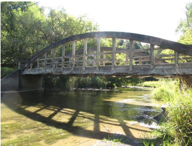
Plate 6: View of north elevation from the west bank.
