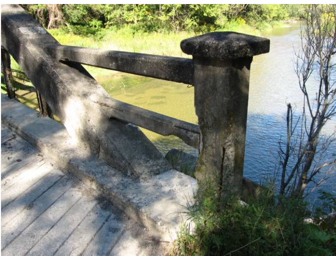
Plate 15: Detail of handrail and end post.
