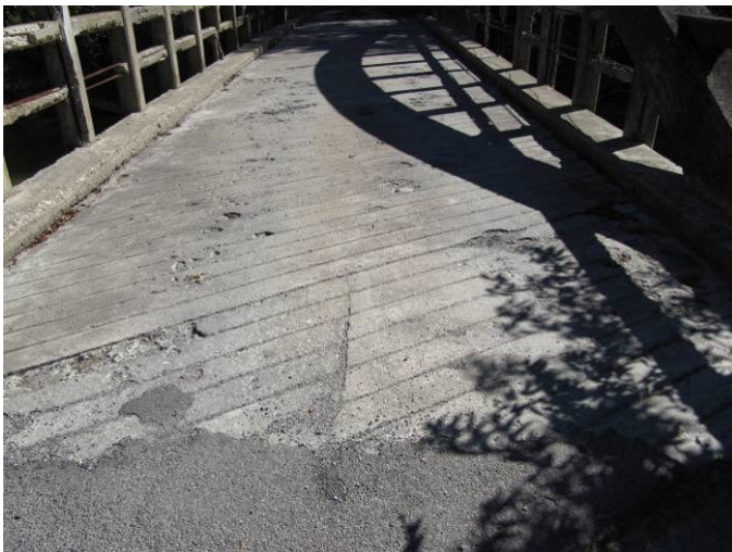
Plate 12: View of the bridge deck.
