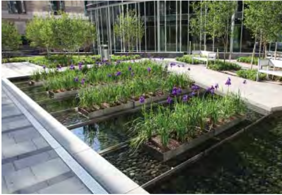
Stormwater Feature on Podium Structure
