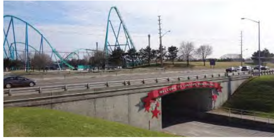
B: Existing Canada's Wonderland underpass
