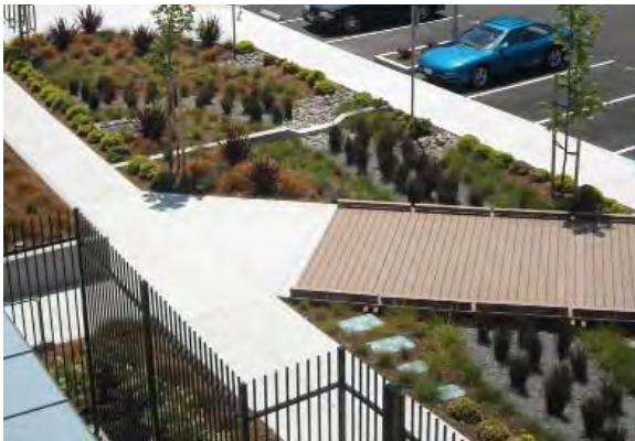
Rain Garden on Grade
