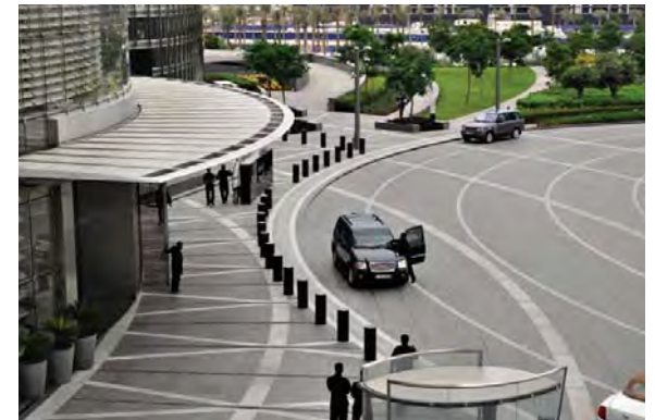
Drop off Entrance Canopy
