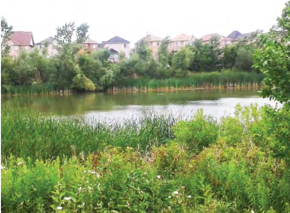
Existing SW Pond North of Precinct
