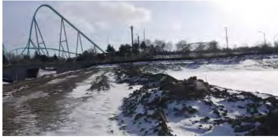
A: View from Future Stormwater Pond
