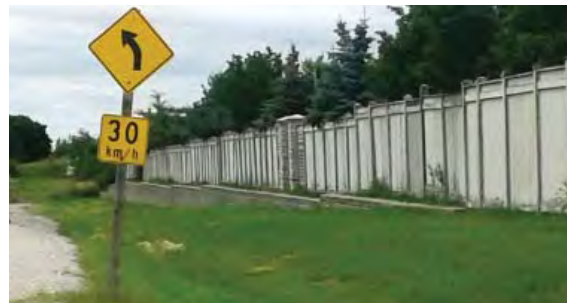
D: Existing Board-on-board fence
