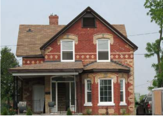
Typical architectural style, quality, and detailing along the Avenue
