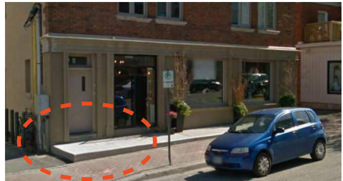
Dead-end conditions to an elevated walkway should be avoided (155 Woodbridge Avenue)
