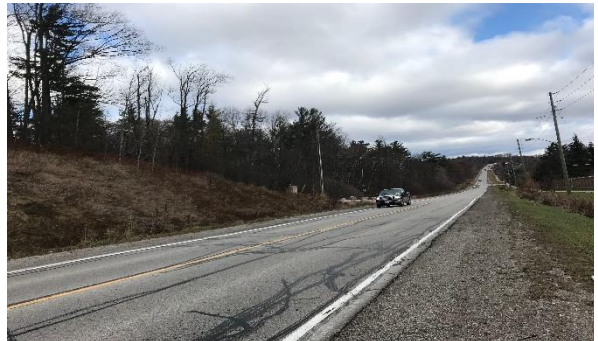
Plate 6: [E] Kirby Road; Area requires test pit survey
