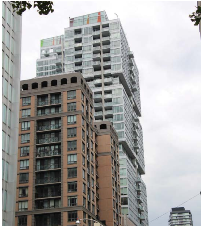
High-Rise buildings should contribute to the City's skyline with attractive and well-defined building components. (Image Credit: Brook McIlroy)
