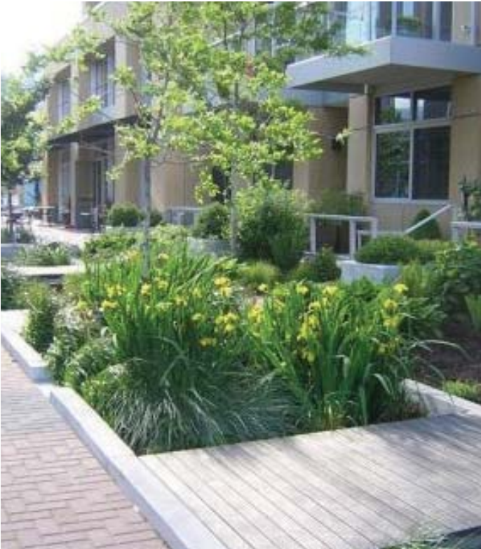
Townhouse units with front yard landscape including stormwater retention areas and tree planting. (Image Credit: Nevue Ngan Assoc.)
