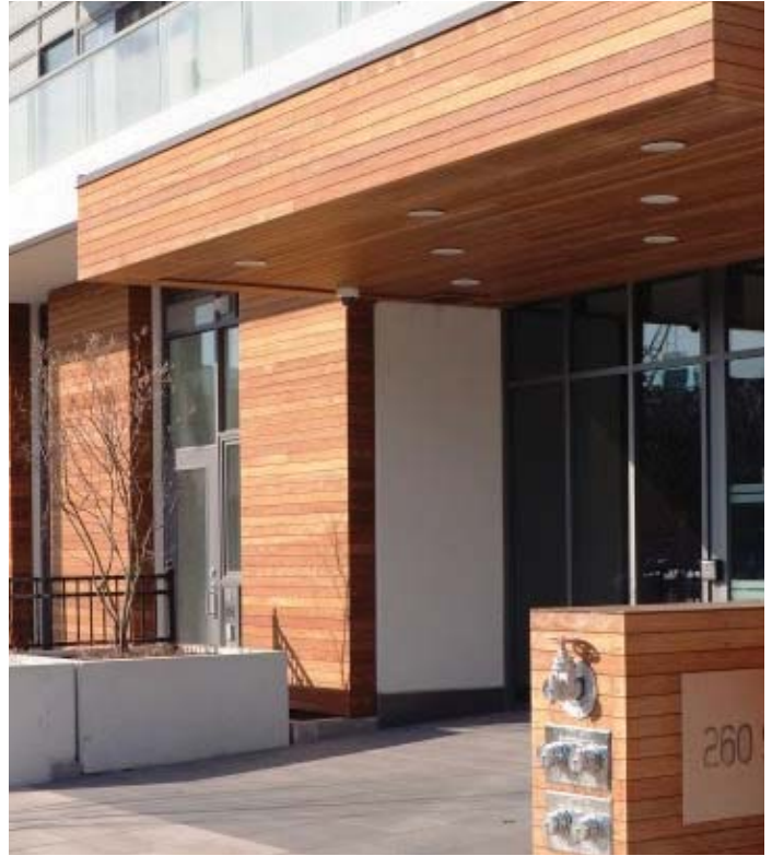
Downlighting integrated into a building entrance. (Image Credit: One Park West, Core Architects, Inc.)
