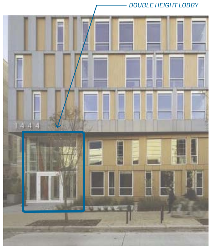
Shared entrance with a double height lobby space and a mix of soft and hard landscape. (La Casa Permanent Supportive Housing / Studio Twenty Seven Architecture + Leo A Daly. Image Credit: ArchDaily)
