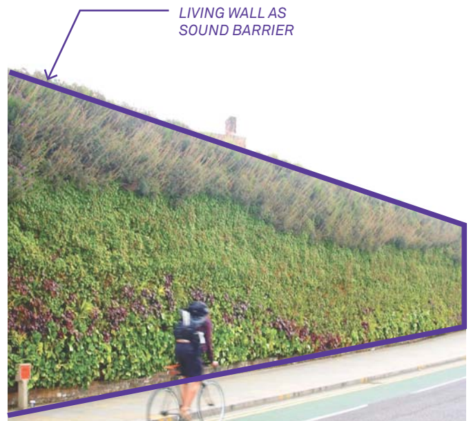
Living sound barriers provide natural amenities and protect other land uses from sound pollution. (Living Wall and King's Cross London. Image Credit: Biotecture)
