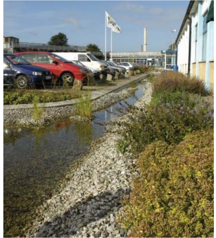
Incorporate L.I.D. measures into site landscape design to manage stormwater on-site. (Image Credit: Brook McIlroy)
