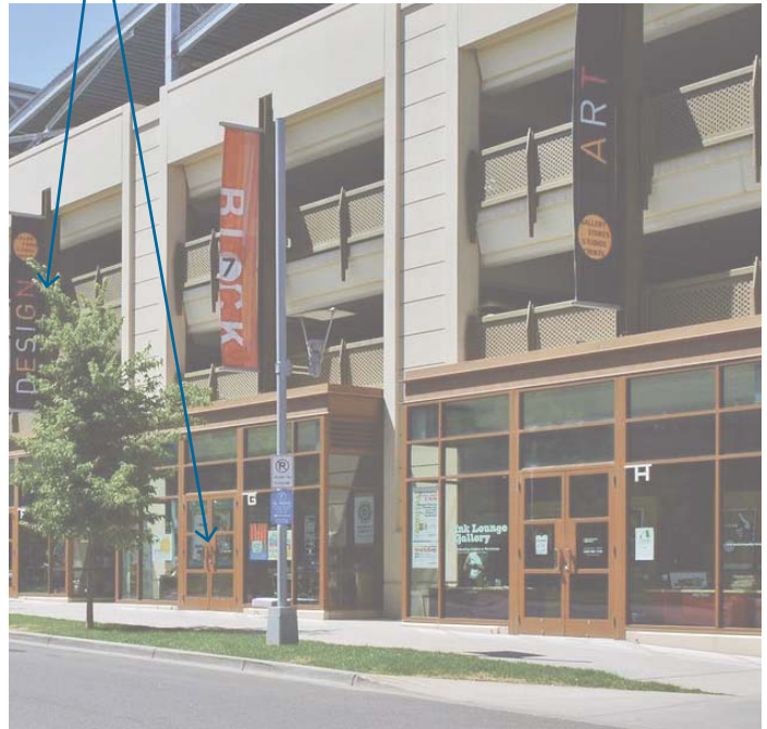
Parking structure wrapped with commercial uses at the ground floor. (Image Credit: Belmar Theatre by Elkus Manfredi, Lakewood, CO. Photo by Chris Whitis courtesy of SitePhocus.com)
