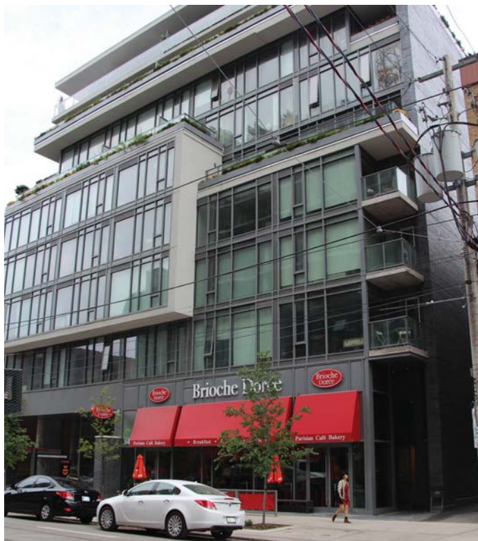
Building articulation helps to address downdrafts and other wind impacts on the pedestrian environment. (Image Credit: Brook McIlroy)
