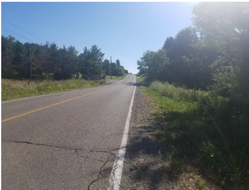
Plate 9: Teston Road; South side of road beyond disturbed ROW requires Stage 2
