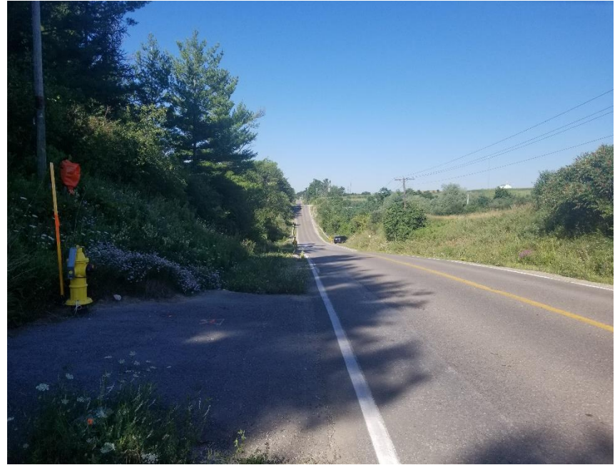
Plate 6: Teston Road; South side of road beyond disturbed ROW requires Stage 2
