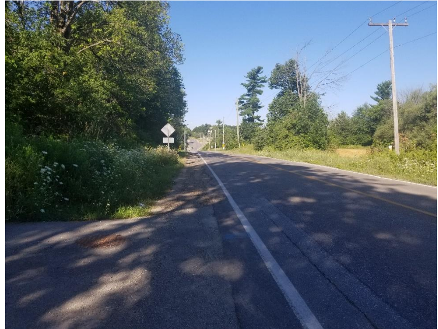
Plate 2: Teston Road; South side of road beyond disturbed ROW requires Stage 2
