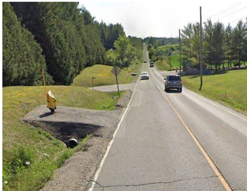
Plate 10: Teston Road; South side of road beyond disturbed ROW requires Stage 2
