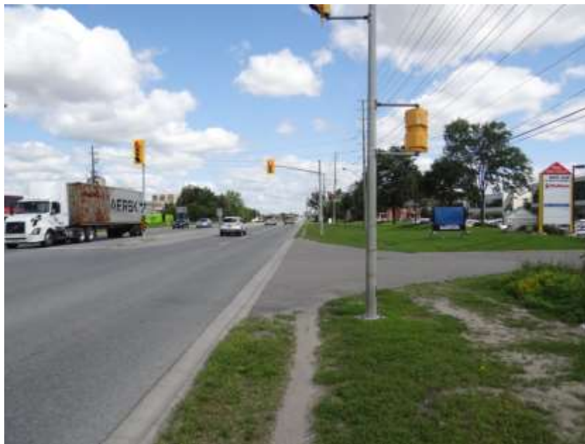
Figure 11: Pedestrian Path on East Approach Looking North
