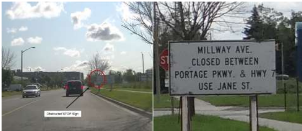
Figure 10: Obstructed STOP Sign in Eastbound Direction
