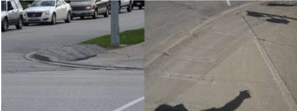
Figure 8 : Encroachment by Heavy Vehicles on Sidewalk
