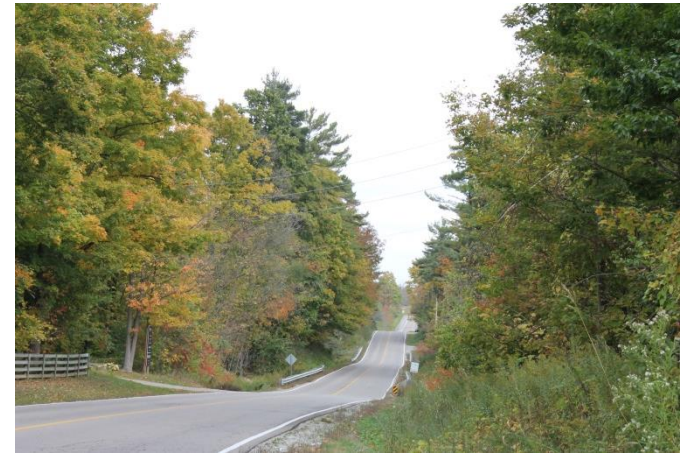
Arterial road (Kirby Road east of Pine Valley Drive)
