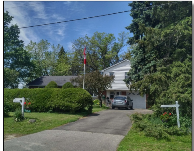
Photo 4: Residence at 11654 Bathurst Street
