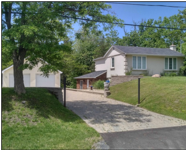
Photo 5: Residence at 11426 Bathurst Street
