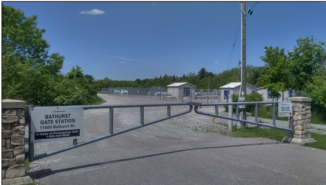
Photo 8: Enbridge Gate Station TransCanada Metre Station adjacent to Bathurst Street
