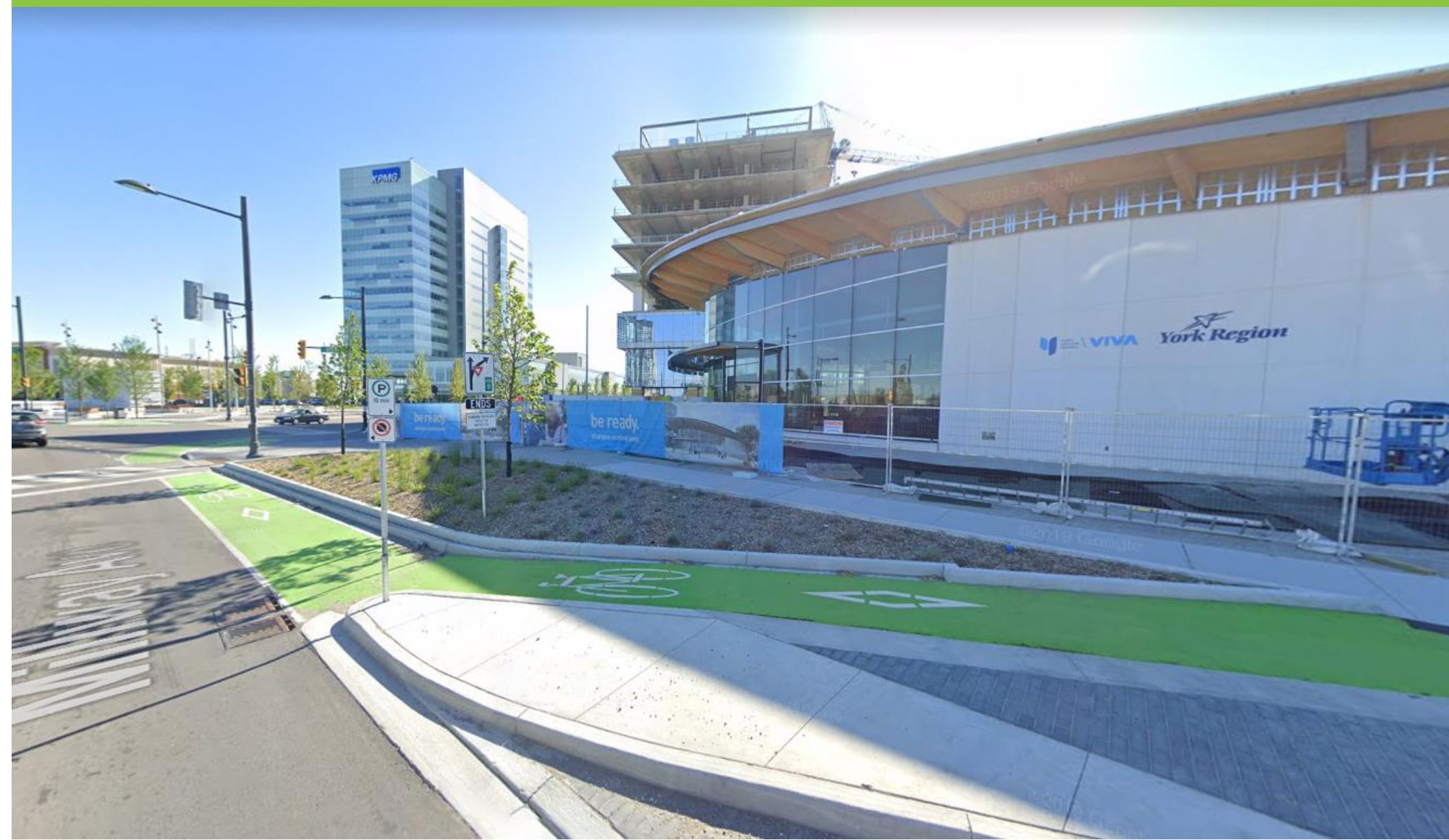
Raised cycle track transition to a conventional bike lane on the approach to an Intersection
