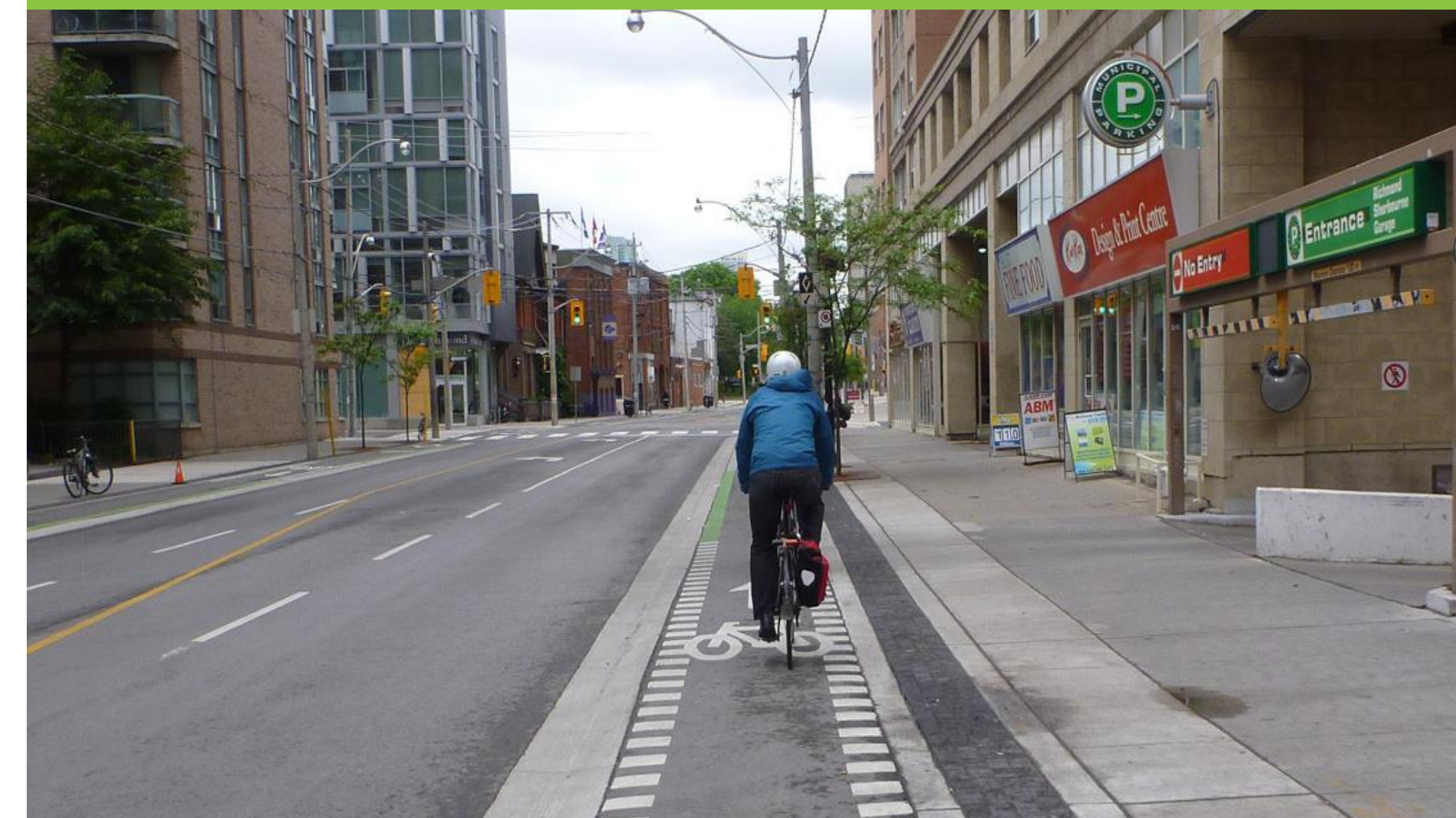
High visibility treatment for cycle tracks at driveways
