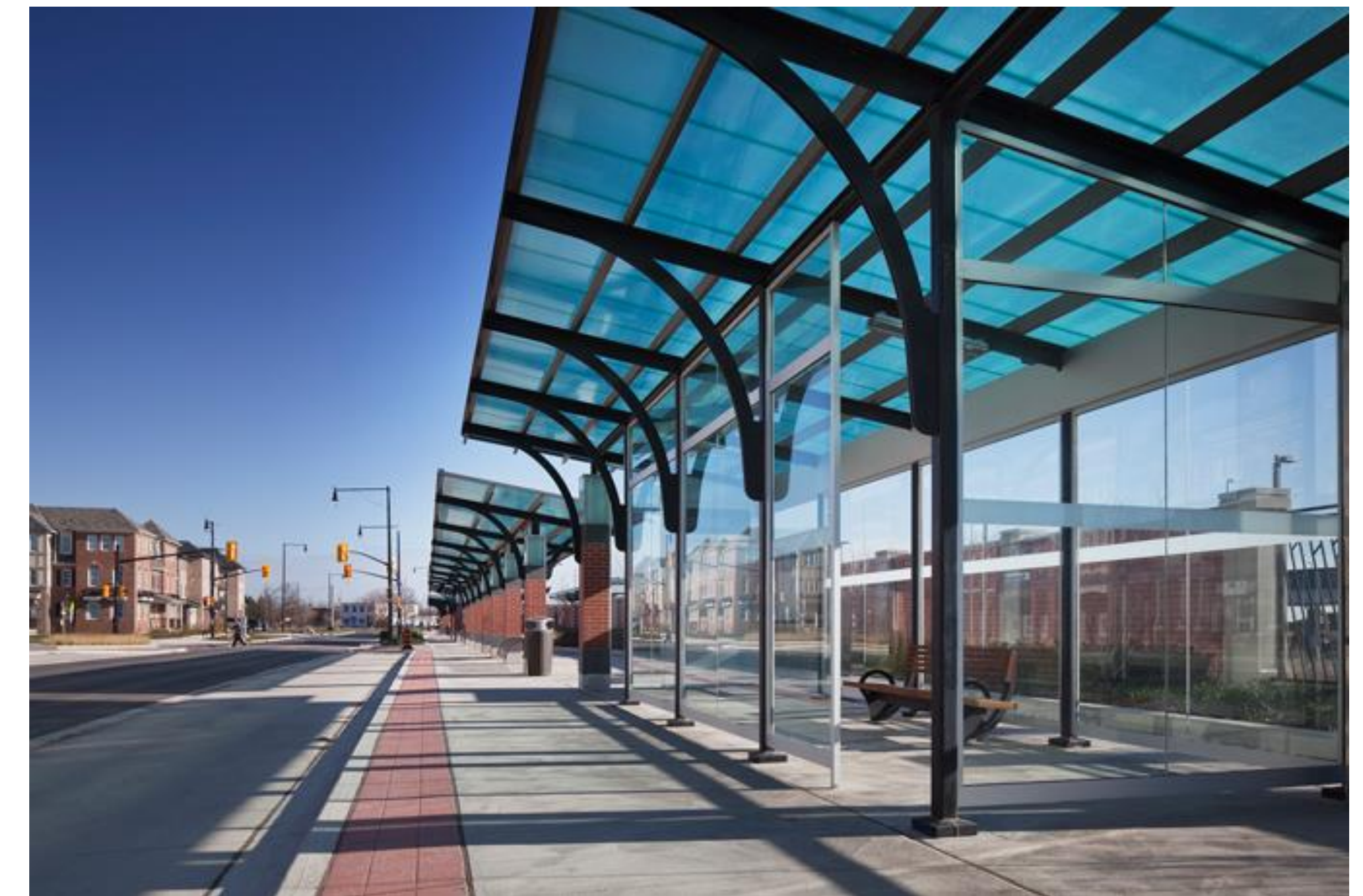
A defining characteristic for Mobility Hubs is the seamless integration of various transportation modes (Mount Pleasant GO Station).
