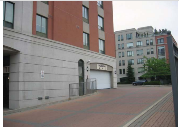
Underground customer parking is not clearly signed from the street.
