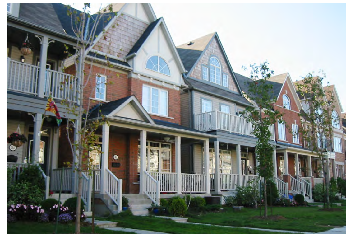
Low to mid-rise residential buildings.
