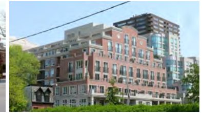
Mixed residential form - stepped back McMurrich Street, Toronto
