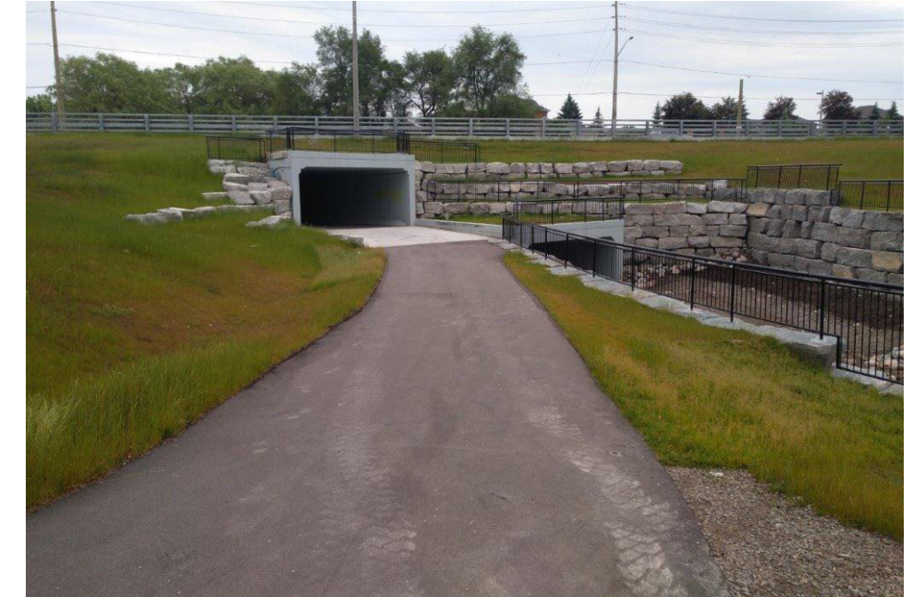
Bartley Smith Greenway and Vaughan Super Trail underpass at Major Mackenzie Drive, constructed in 2019
