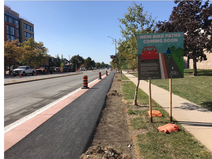
Cycle tracks under construction along Clark Avenue (2020)
