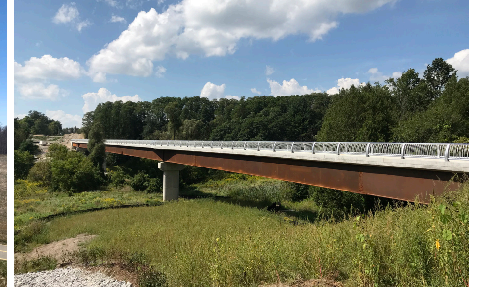
Purpleville Creek pedestrian bridge at Pine Valley Drive and Teston Road
