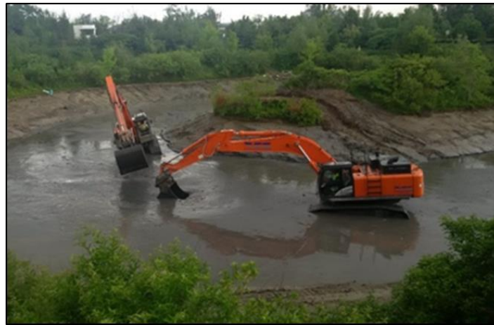
Larissa Stormwater Pond
