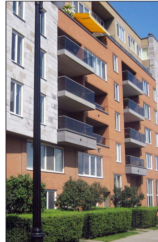
Fig. 2.3.3c Mid-rise building frontage.
