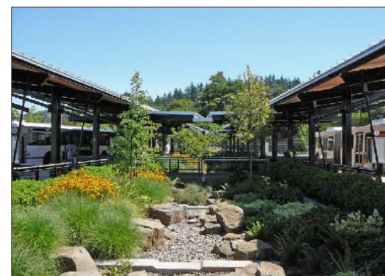
Fig. 2.2.8a Rain garden in Portland, OR.
