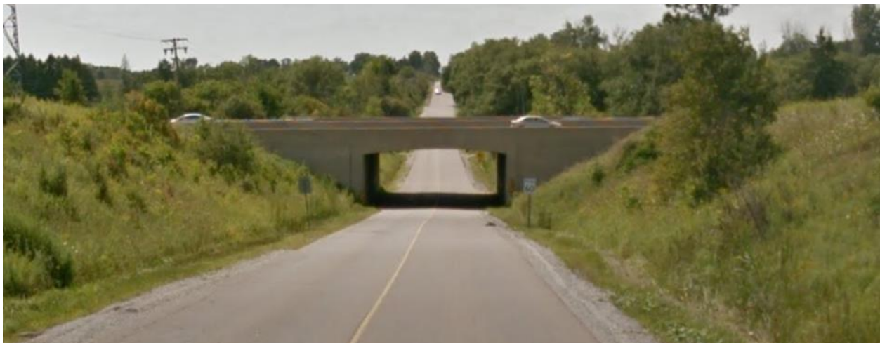
Exhibit 4-4: Kirby Road under Highway 400 Source: Google Maps
