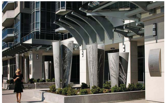
Artist: Linda Covit. An example of a private sector, percent for art project that enhances the streetscape while providing detail and interest for the building that the artwork was commissioned for.
