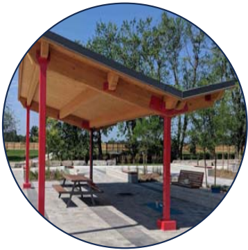
1 Feature shade structure. Focal point within the park
