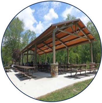
1 Replacement Shade Shelter for Smaller Group Gatherings
