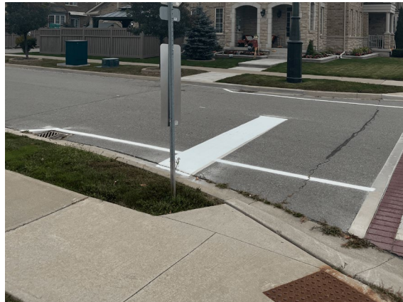
Curb Extension at Barons St/Richler Ave
