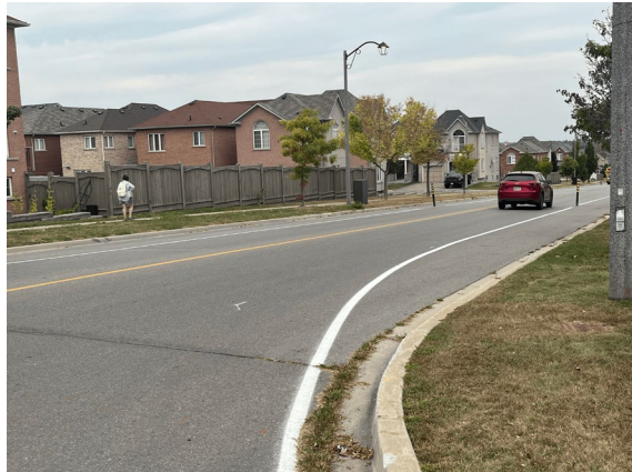
Edge Lines on Peter Rupert Ave
