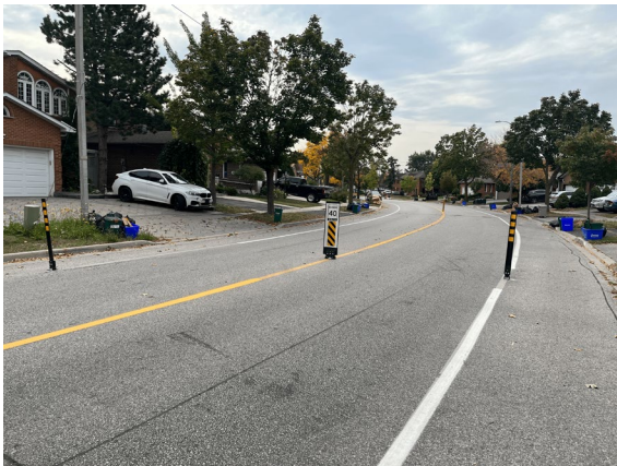
Centreline Flex Post combined with Bollards. on Conley St
