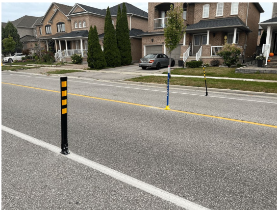
Slow Down School Zone Flex Post combined with bollards on Napa Valley
