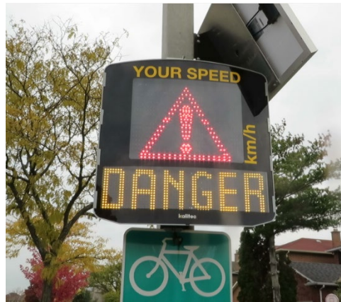
Radar Message Board at Conley St
