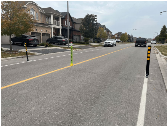
Slow Down School Zone Flex Post combined with bollards on Peter Rupert Ave
