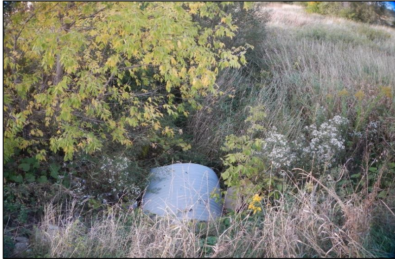
Figure 3-14: Upstream View of Drainage Feature 6 from Teston Road (September 2019)
