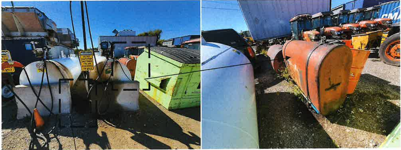
ASTs including two diesel ASTs with the associated fuel dispenser to the south of the barn and maintenance shop at 11244 Keele Street, the eastern portion of the subject site (looking west)
