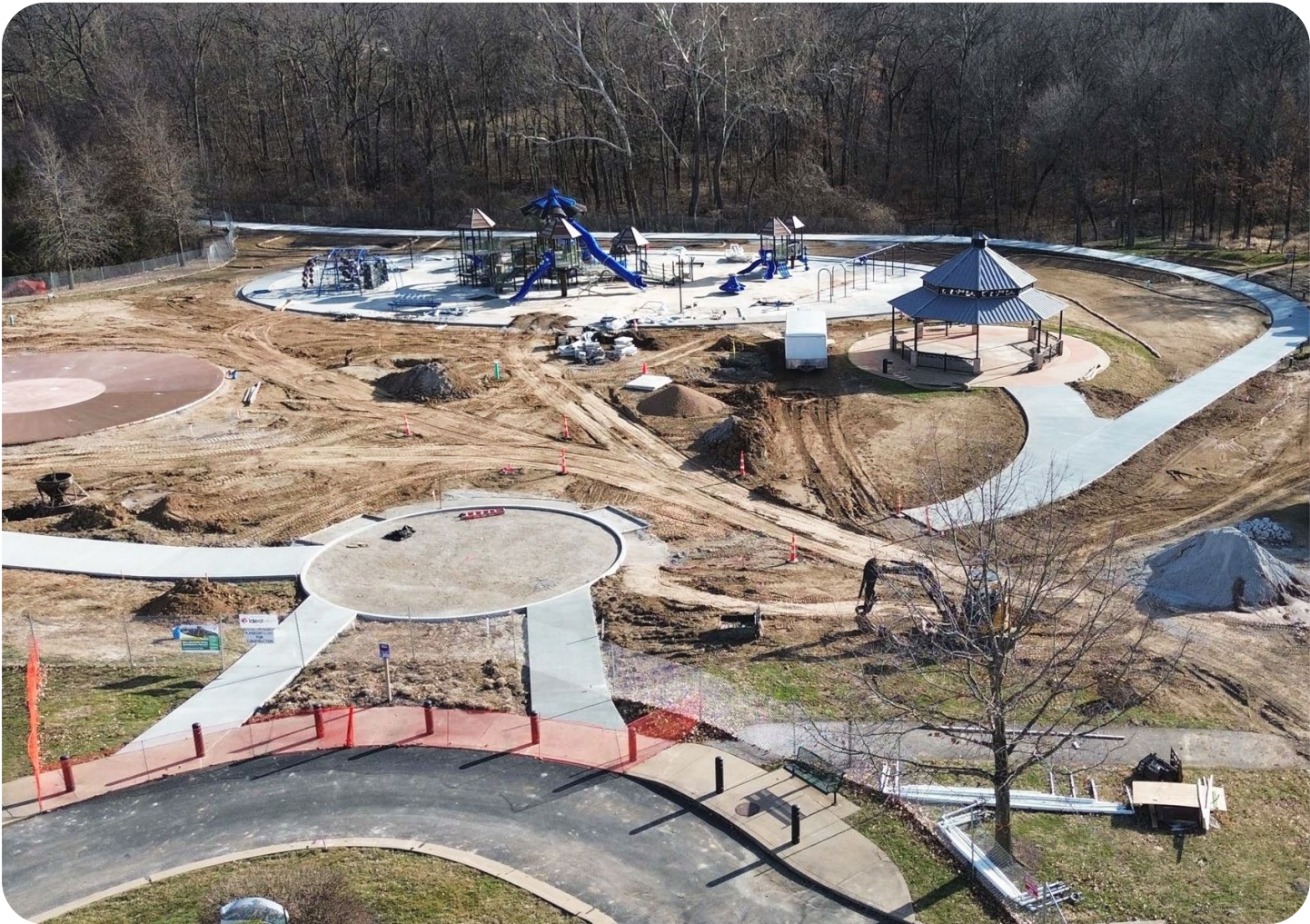
Figure 93 - Millennium Park, Creve Coeur, Missouri
