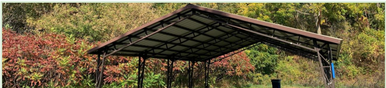
Image 19: Existing shade structure at Doctors McLean District Park
