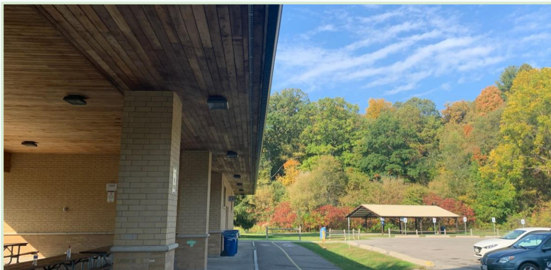
Image 10: Existing shade structures at Doctors McLean District Park
