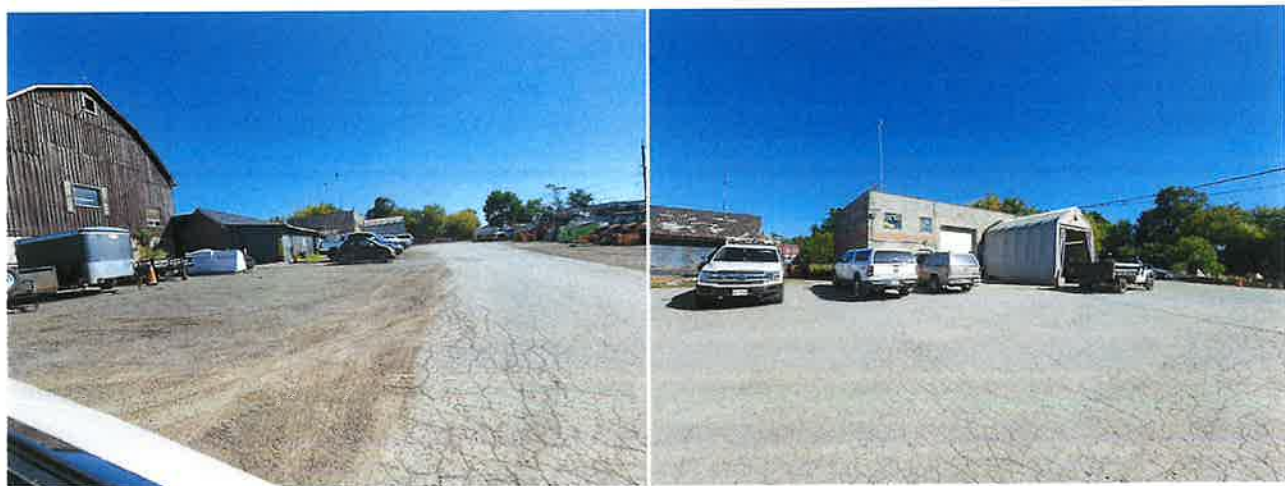
General view of construction and landscaping machineries storage (left) and office and maintenance shop located at the central portion of 11244 Keele Street (looking south and east, respectively)
