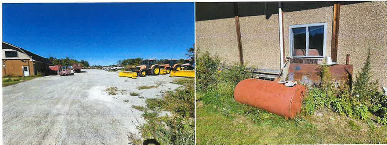
General view of construction company (left) located at the northeast corner of the western portion of 11244 Keele Street, at the central portion of the subject site (looking north) and 3 ASTs (right) located to the west of the commercial building (right – looking east)
