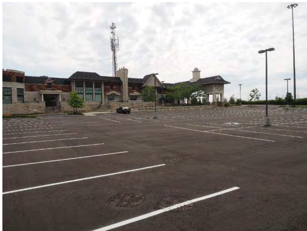
Image 7: View of disturbances associated with paved area, utilities, and extant structure.
