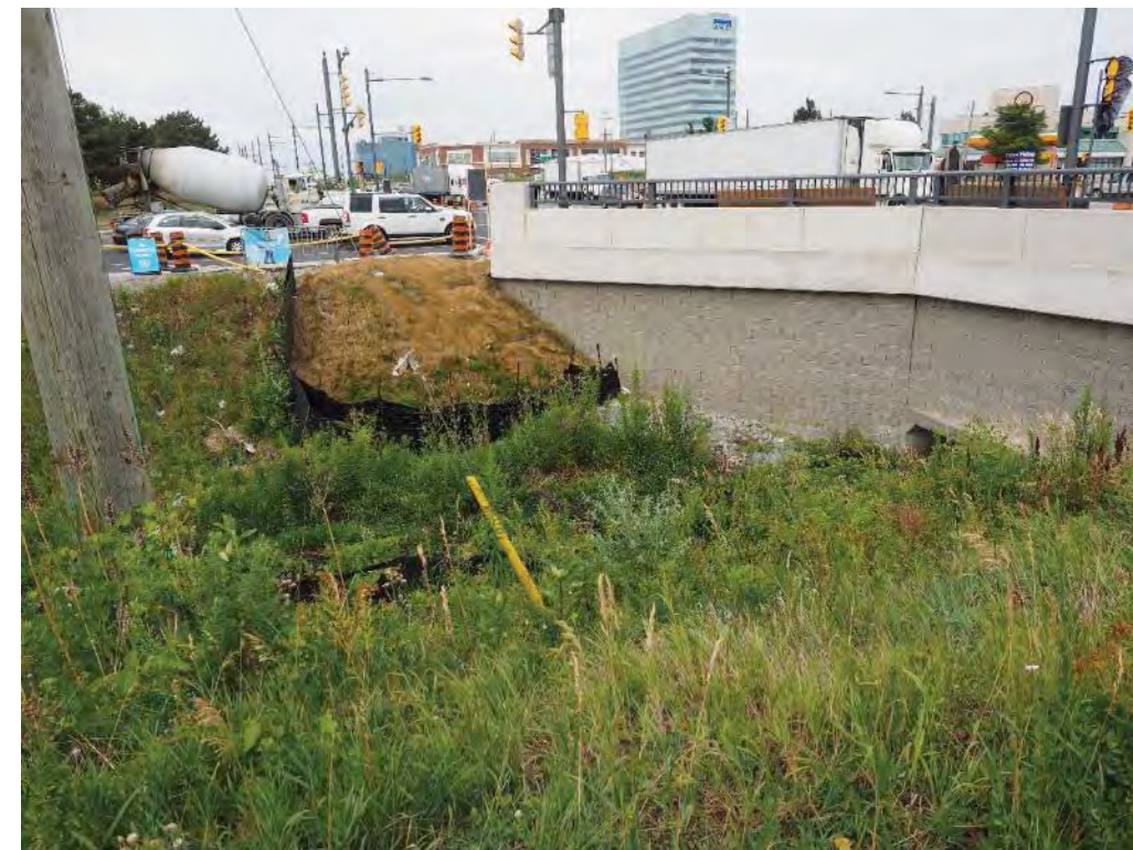
Image 12: View of disturbances associated with culvert and utilities.
