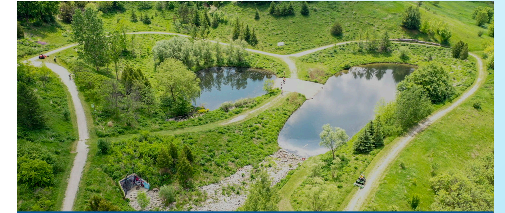
150 stormwater management ponds
