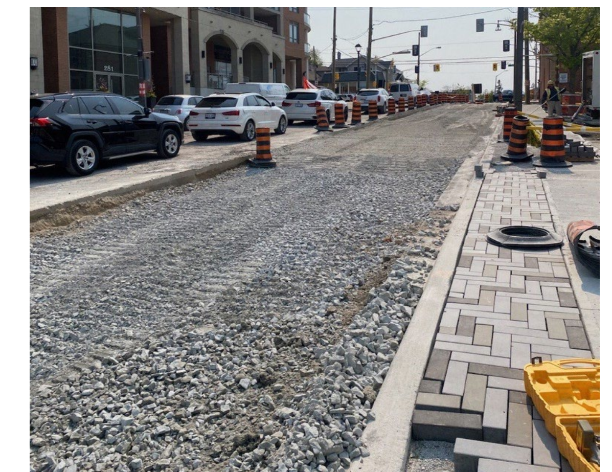
Typical paver stone interlock installation
