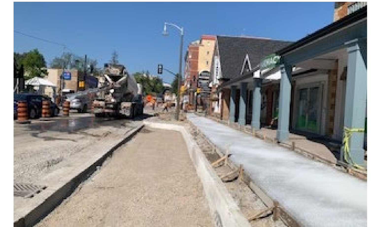
Typical streetscaping construction of curb and sidewalk
