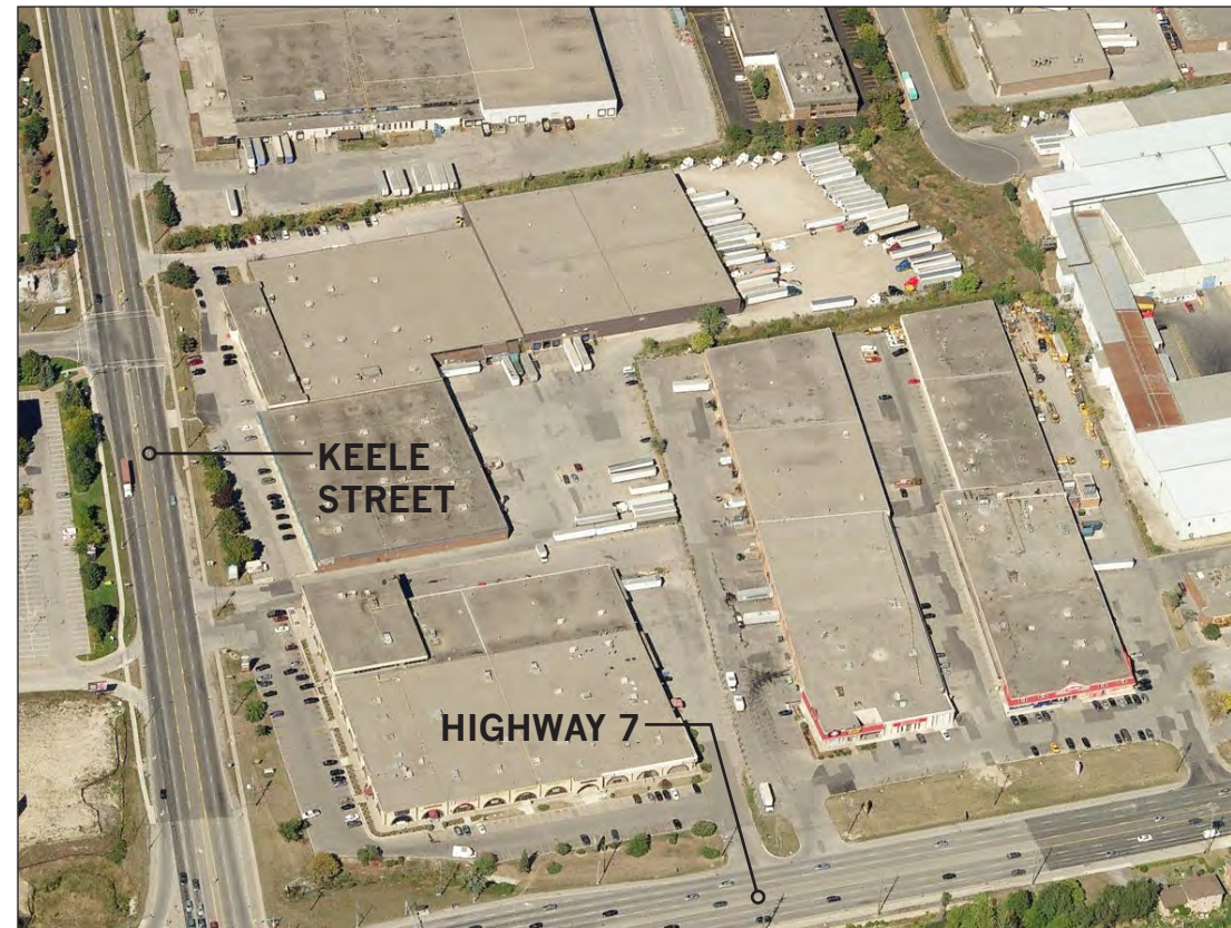
Figure 2.1.3 Detailed aerial view of typical existing conditions within the study area.
