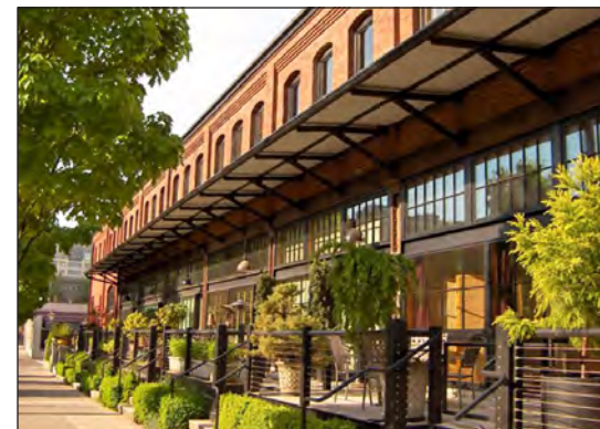
Fig. 2.3.3b Raised street front patio.
